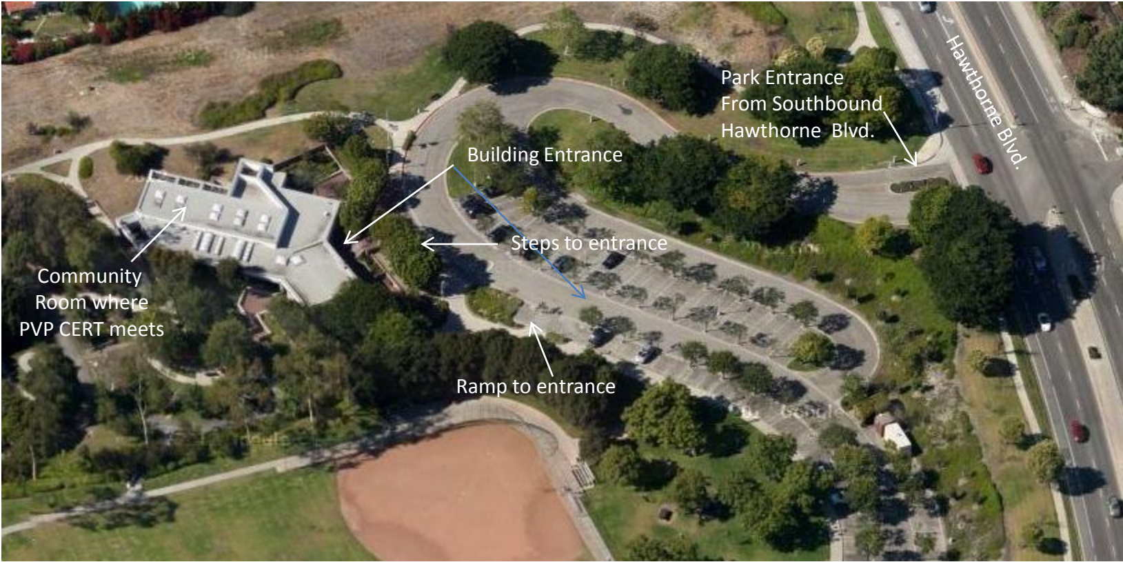
Credit for aerial view: Google Maps
